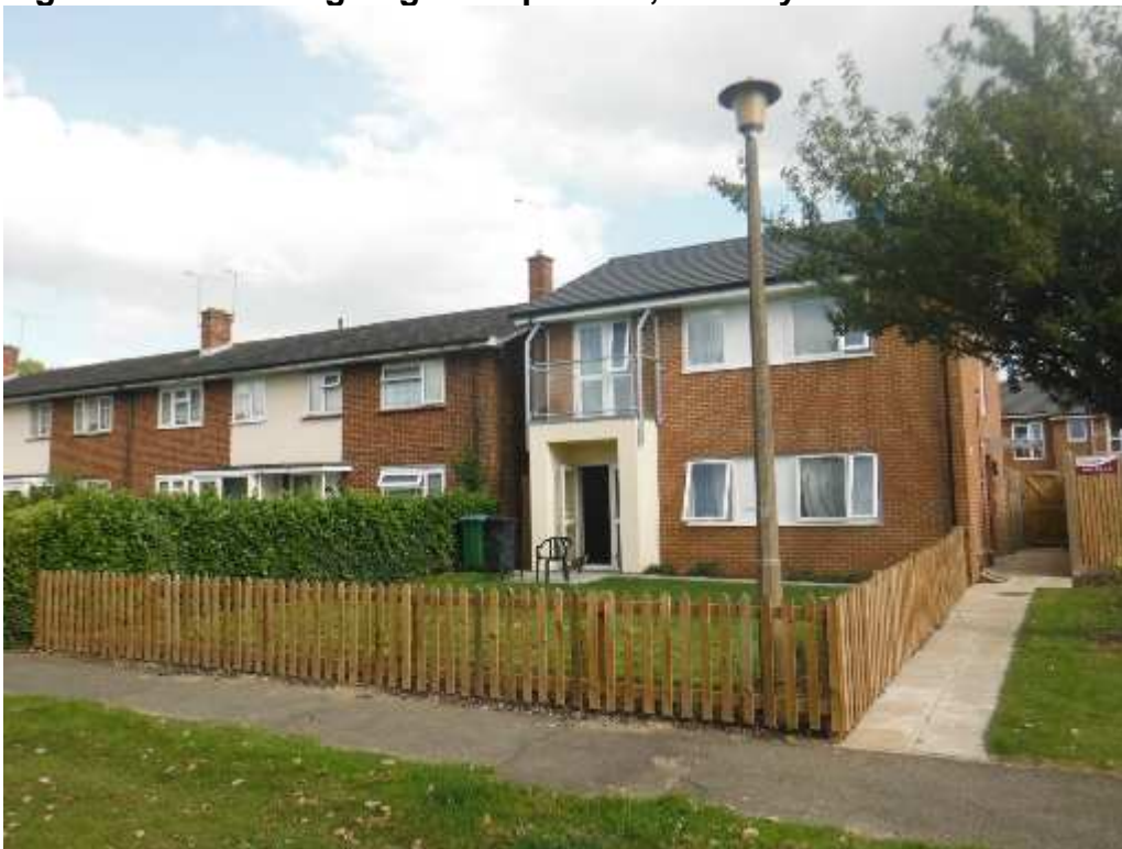
Figure 9-2: Former garage compounds, Croxley View
